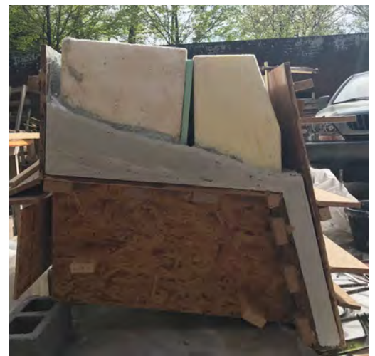
Formwork Disassembly
